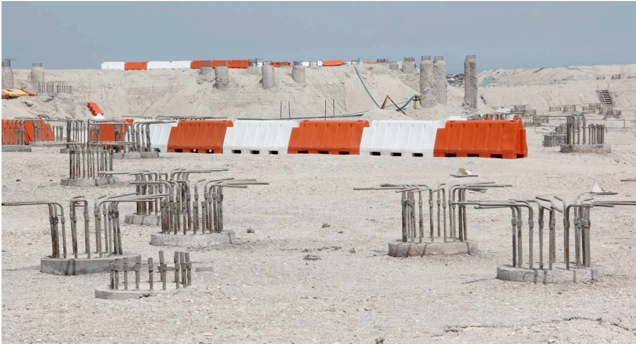
Pilings and earthwork at the Guggenheim site, 20th March 2014
